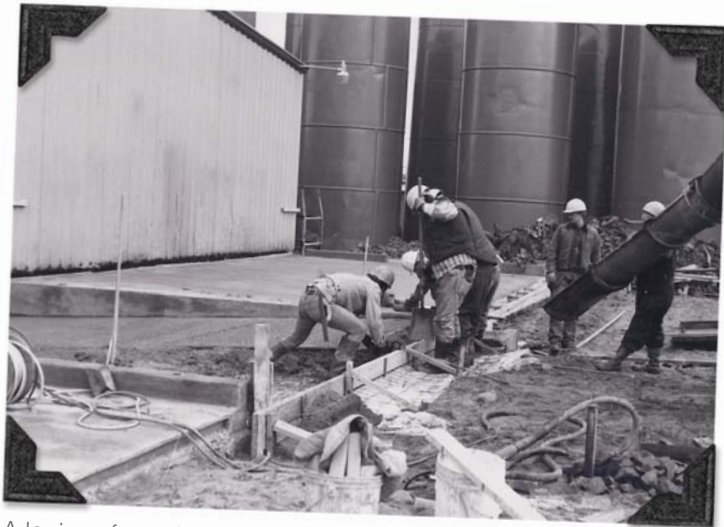
A legion of passionate AMSOIL Dealers sparked explosive company growth, requiring construction of new bottling lines, holding tanks and other infrastructure.
